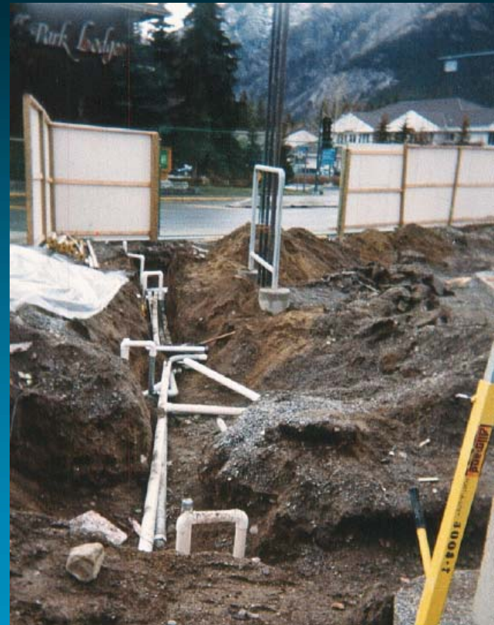
Piping near south property line and west of building
