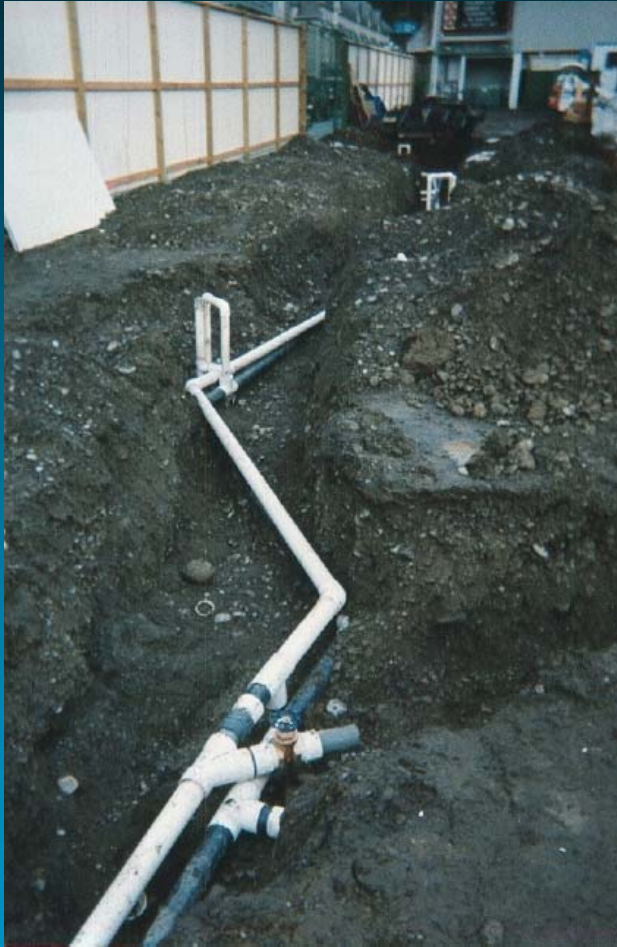
Piping north of new pump islands
