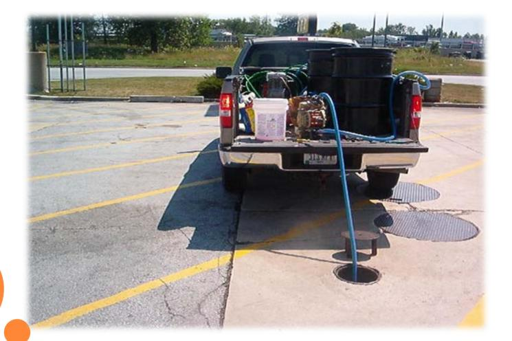
Injection of Surfactant Solution Into UST Area Via Two (2) Observation Wells (July 30, 2008)
