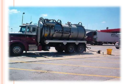
Power Vacuum System Operating At UST Extraction Wells After Surfactant Injections:
