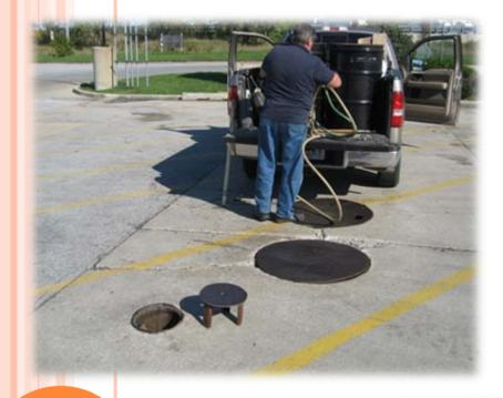
Injection of *Ivey-sol*® Surfactant Solution At UST Area Via Two (2) Observation Wells October 9, 2008
