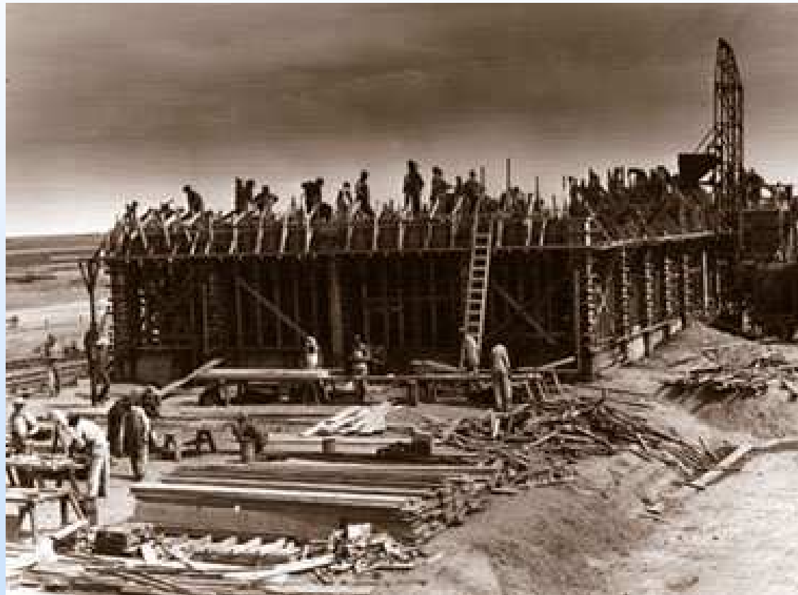
Construction of the first chemical weapons manufacturing facility at the Rocky Mountain Arsenal, 1942 (U.S. Army photograph)
