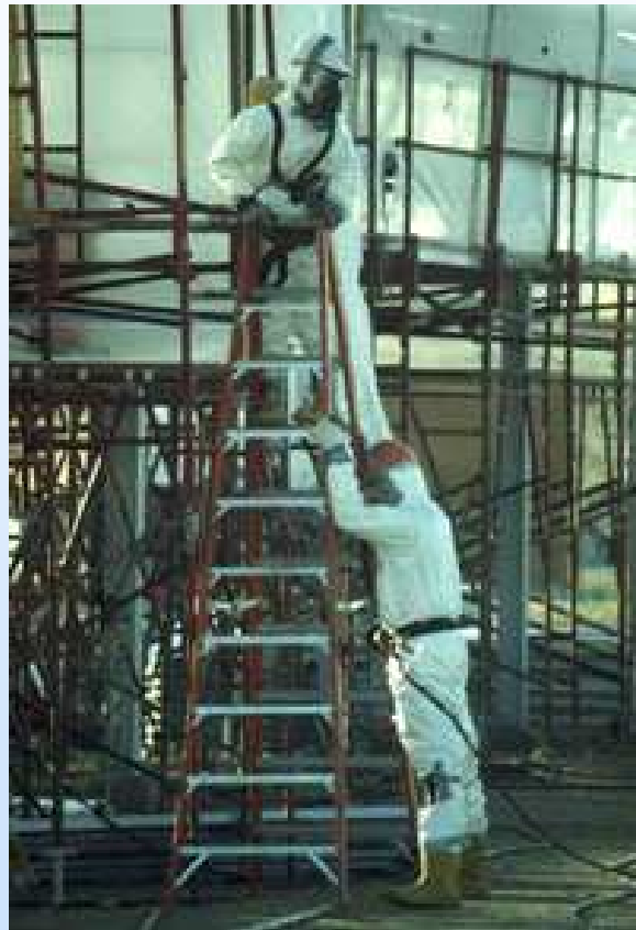
Asbestos abatement in South Plants (U.S. Army photograph)
