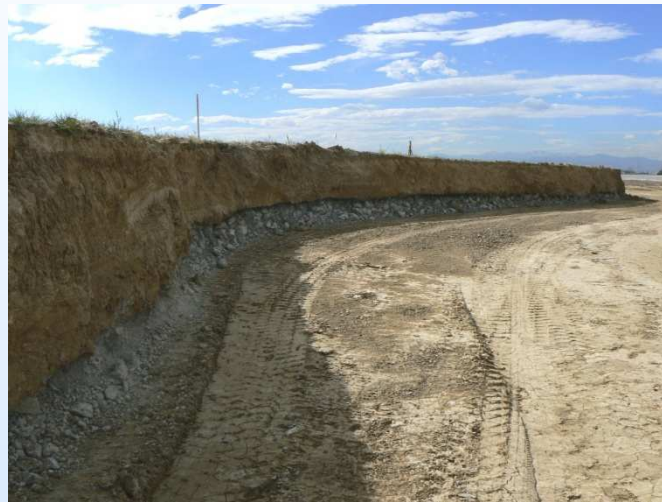
Cross section through the Shell RCRA-Equivalent Cover. 18 inches of BBM is overlain with a geotextile and 4 feet of soil (EPA field oversight photograph). Cross section of RCRA-E Covers (TetraTech EC 2008)
