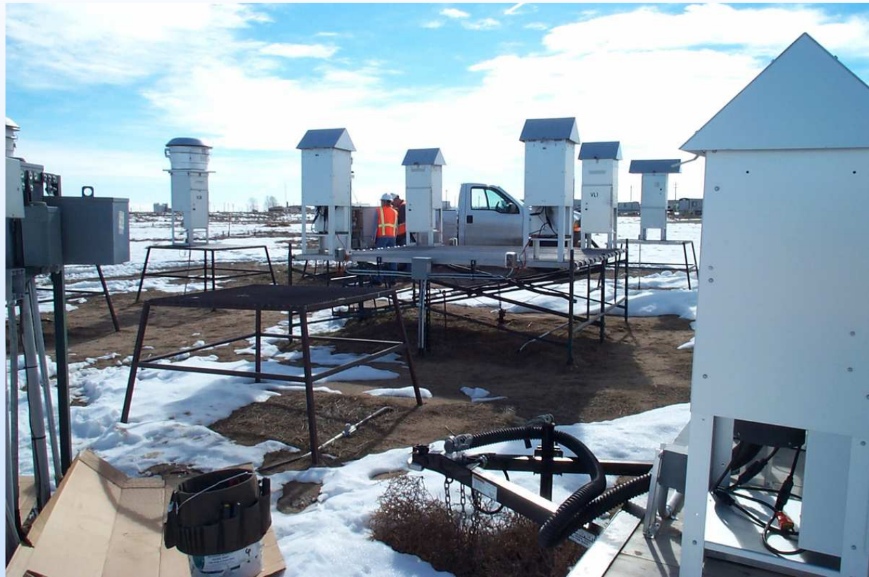
Air monitoring station for chemical emissions at RMA (EPA field oversight photograph)
