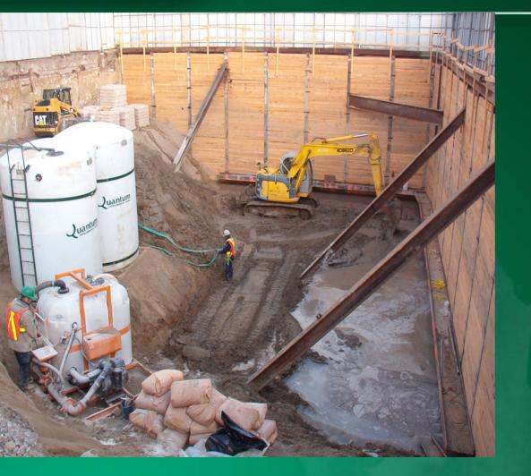
Slurry Slot / Concrete Backfill Barrier Wall
