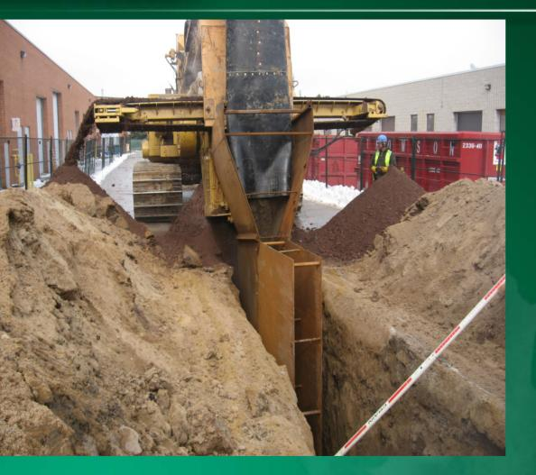
Trenching machine simultaneously excavates trench and installs backfill media
