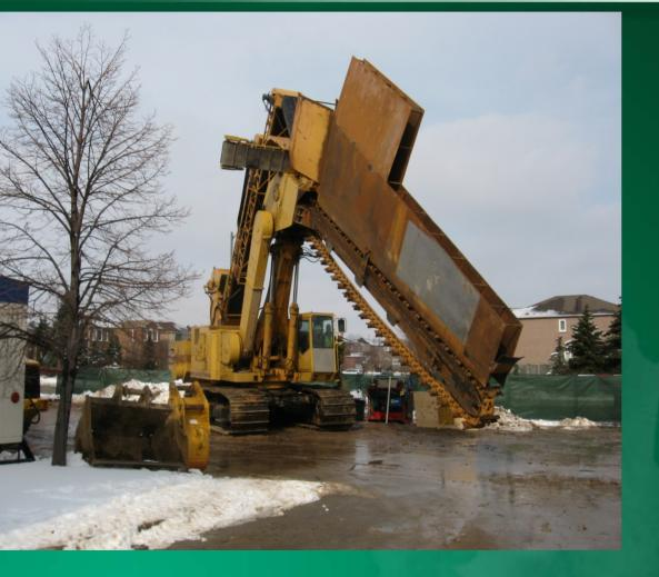
Trenching machine simultaneously excavates trench and installs backfill media
