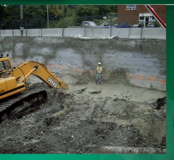
Slurry Slot / Concrete Backfill Barrier Wall
