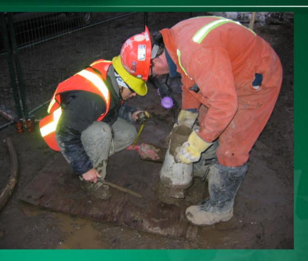
Field Preparation of Soil-Bentonite Admixture (Trench Backfill)
