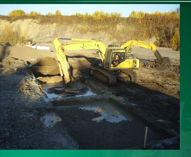
Field Preparation of Soil-Bentonite Admixture (Trench Backfill)
