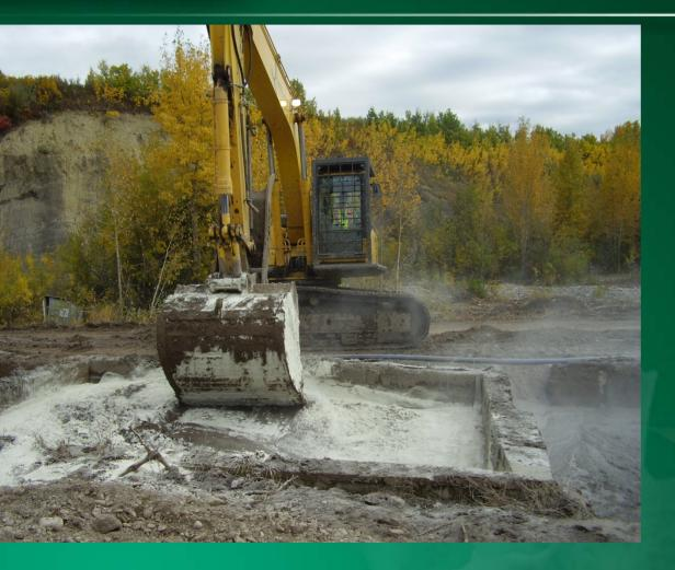
Field Preparation of Soil-Bentonite Admixture (Trench Backfill)
