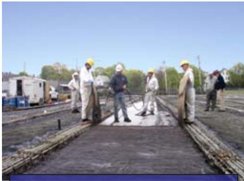
Former Manufacturing Facility
