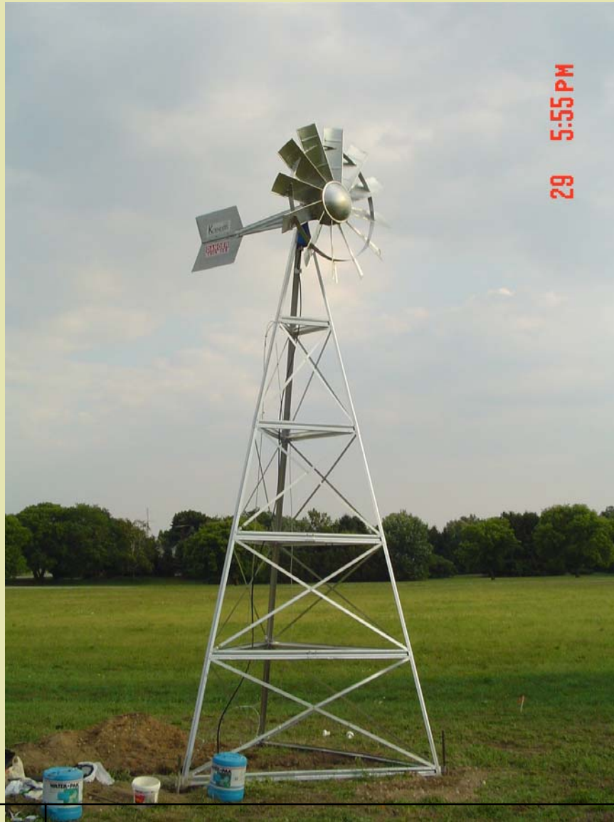
Case Study 2: Windmill and Air-Sparge system installation.
