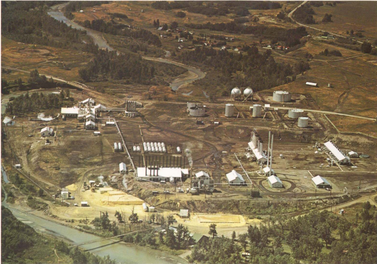
PLANT SITE — TURNER VALLEY, ALBERTA NATURAL GAS PROCESSING AND PURIFICATION PLANT
