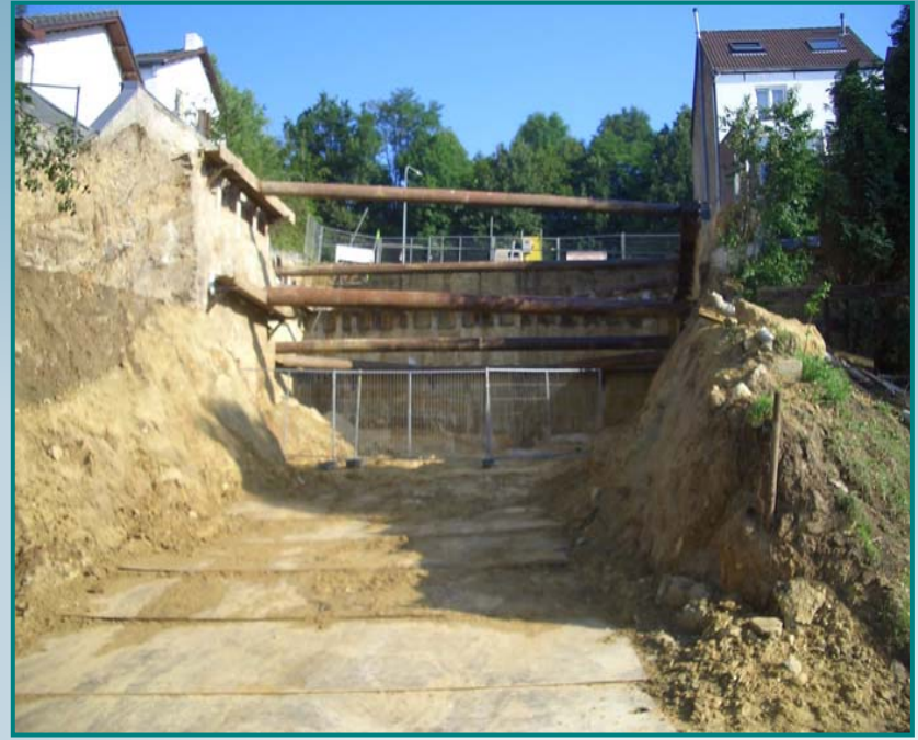
AFTER (excavation completed)
