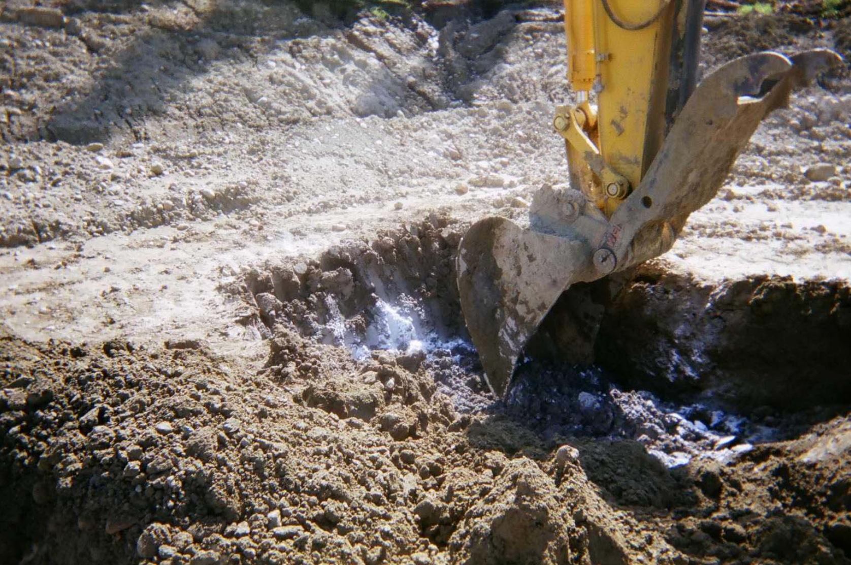
Blending EDTA into the soil-waste mix
