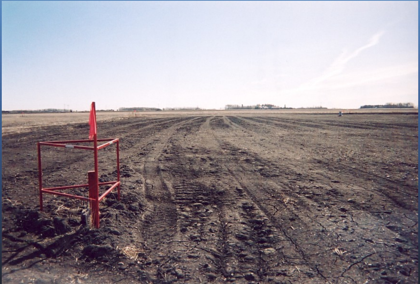
After Backfilling and Leveling
