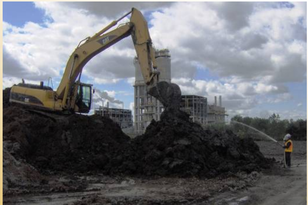
Pumping of the fluid to the soil
