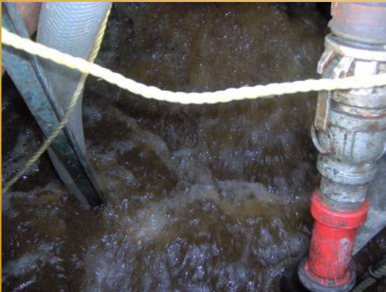
Aeration and mixing
