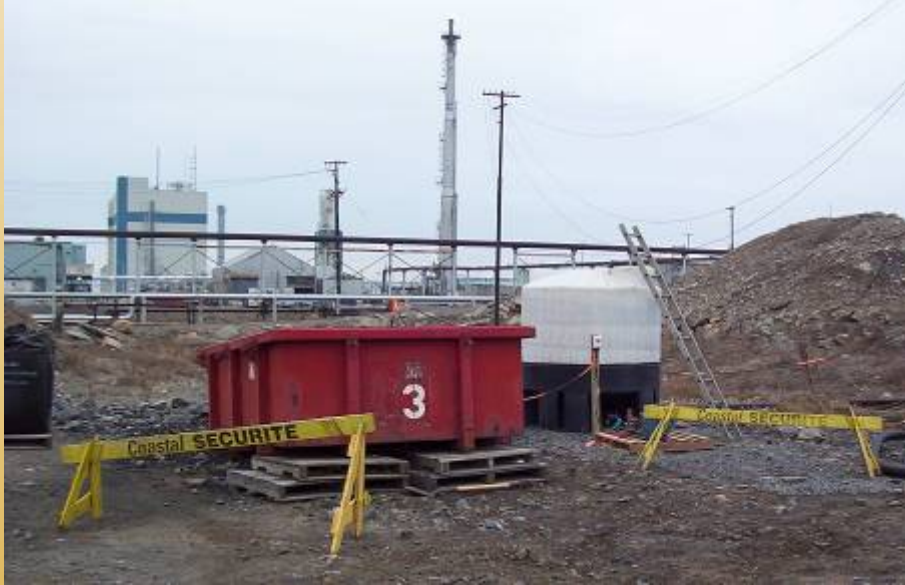
Sludge box and bioreactor for seeding of soil
