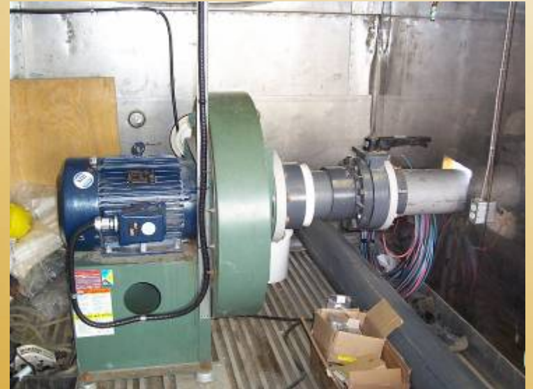
Blower to circulate air and increase temperature above the dew point
