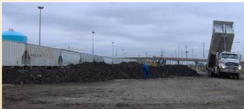
Delivery of the soil at the K-1 site for construction of a berm for a visual barrier
