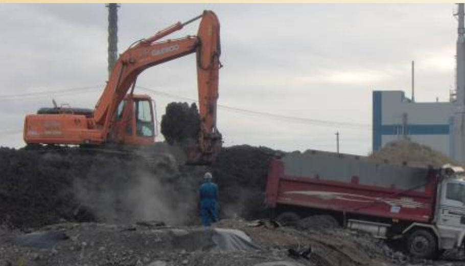
Loading of treated soil
