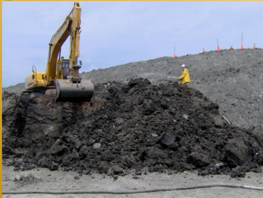
Pumping of the fluid to the soil
