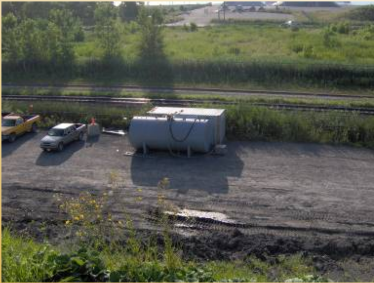
A bioreactor is used to grow an indigenous microbial population
