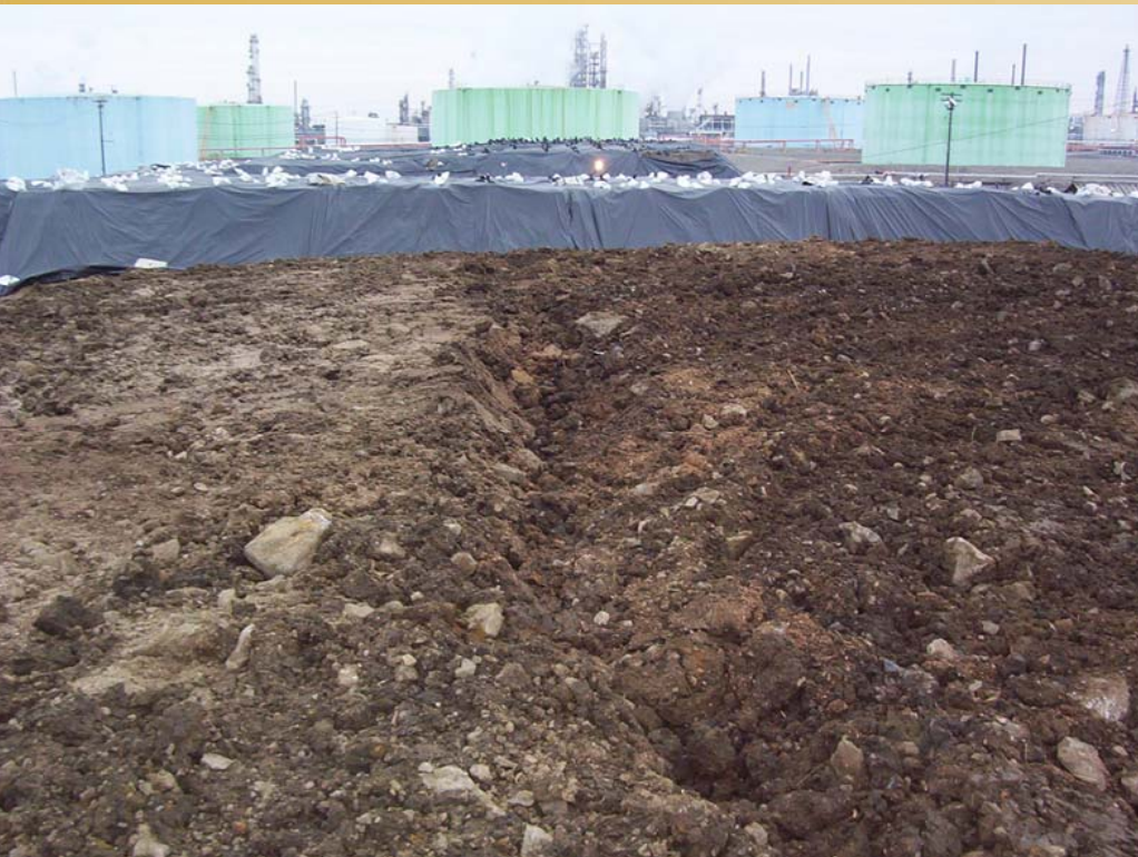
Soil after conditioning with amendments and mechanical mixing
