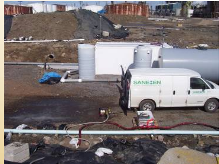
Pumping to well points in the biopile
