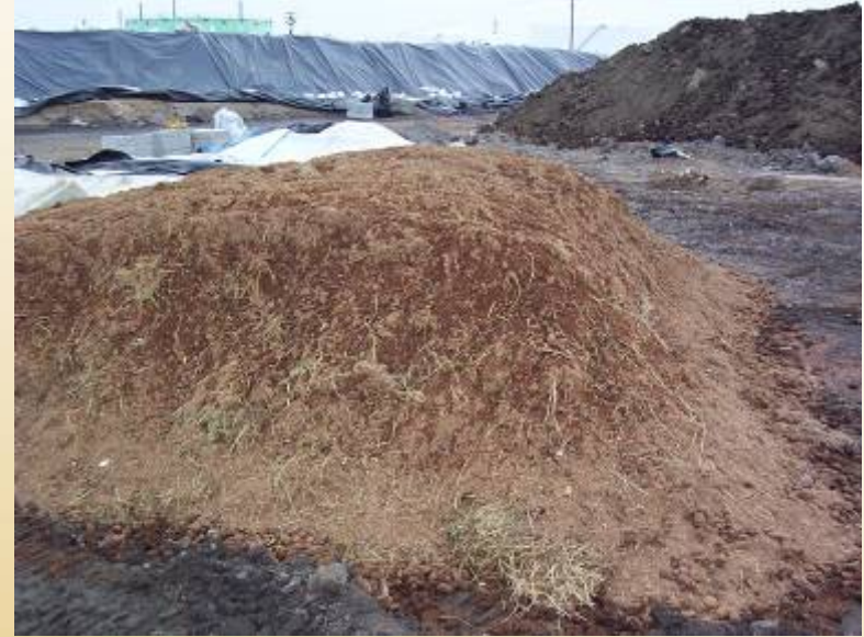
Biomass amendment for bulking of soil
