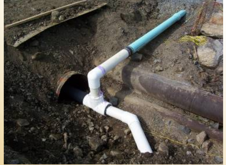
Connections to the air treatment system
