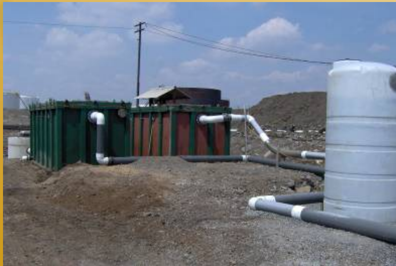
Biofilters and an adsorption filter for the treatment of air
