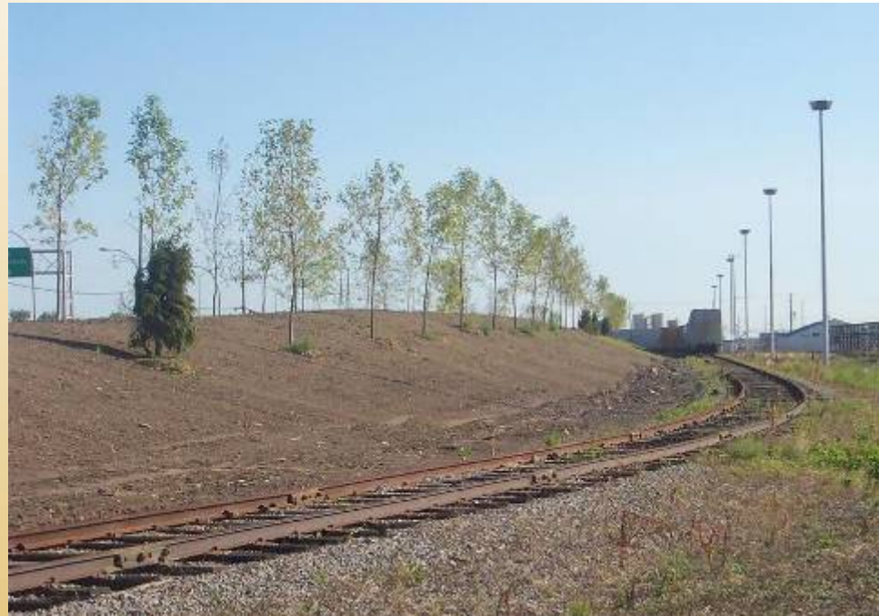
K-1 berm along the Metropolitan highway
