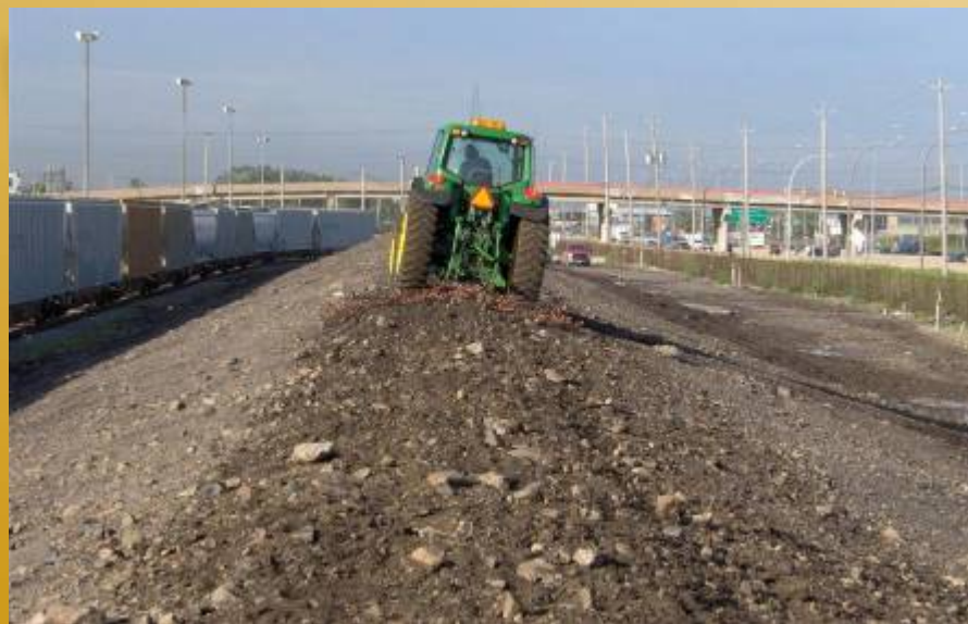
Profiling of the berm
