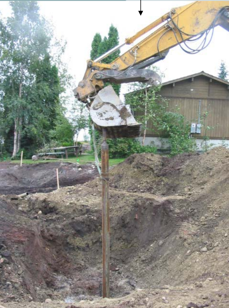
Casing Removal
