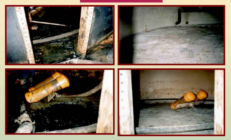
Tank Cleaning Applications Before & After Ivey-sol® Cleaning
