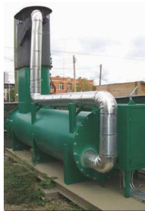
Catalytic Oxidizer (Incinerator) for Off-gas Destruction
