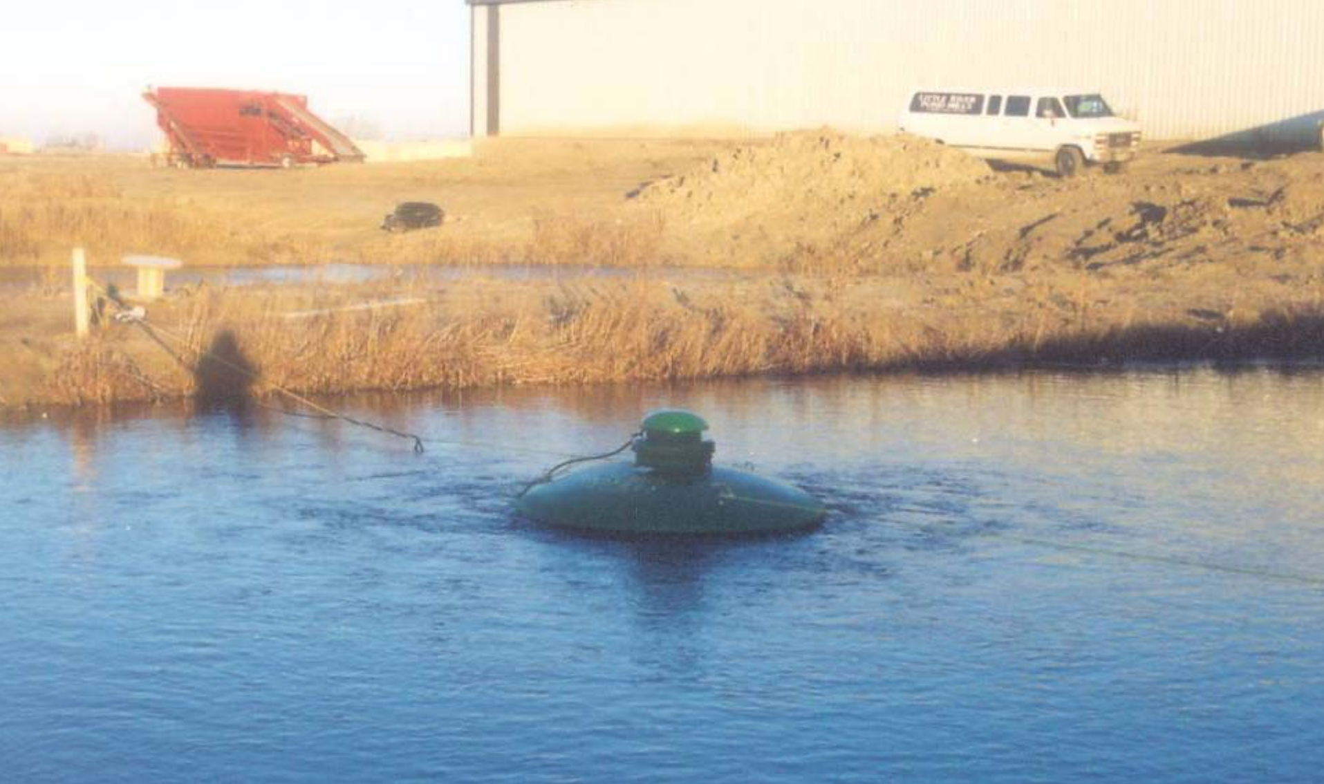
Little River Pond Mill ® circulator installation for treatment of potato processing waste water – Alberta, Canada
