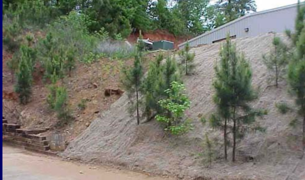
Jute Matting Installation
