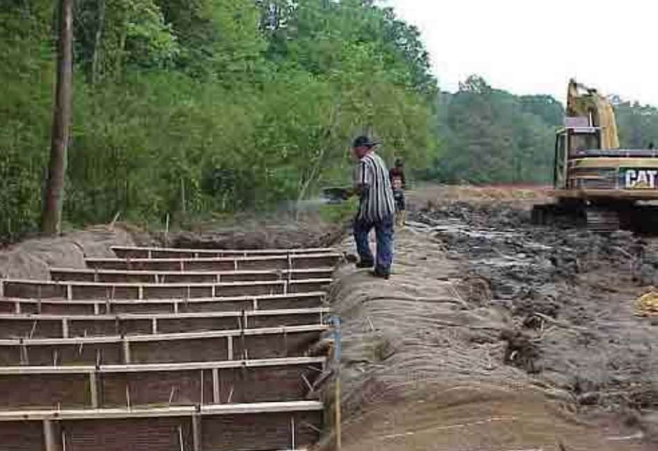
Baffle grid with polymer, used to reduce turbidity of discharged water
