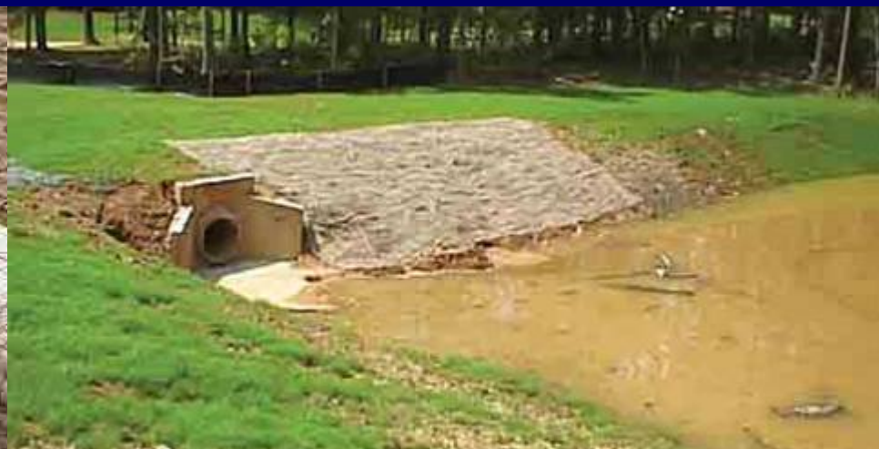
Soft Armoring with polymer along a slope to prevent further erosion
