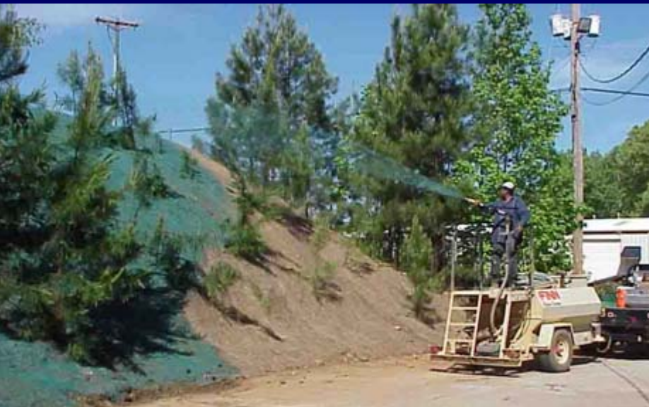
Hydro Mulch Application with APS Blended PAM and Grass Seed
