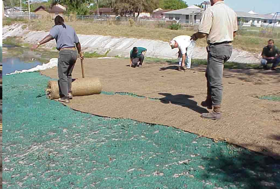
Soft Armoring with polymer over blown mulch using jute woven mat
