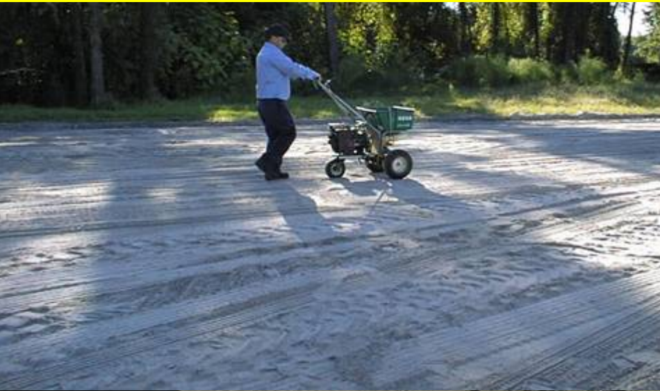
50 lbs Polymer Powder Applied With Fertilizer Spreader
