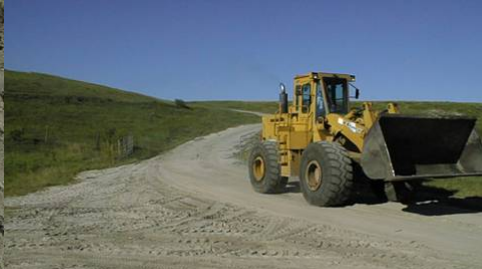
Dust Controlled With 1 Daily Water Wagon Application For 45 Days
