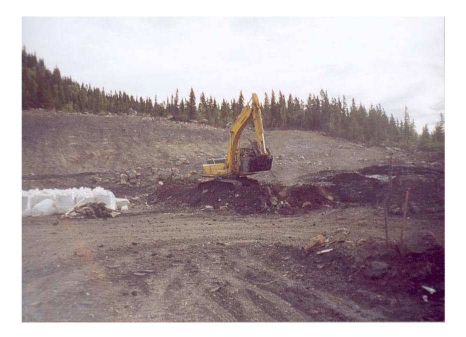
Water and Portland Cement were then added and the amalgam was mixed for 20 hours with a common backhoe
