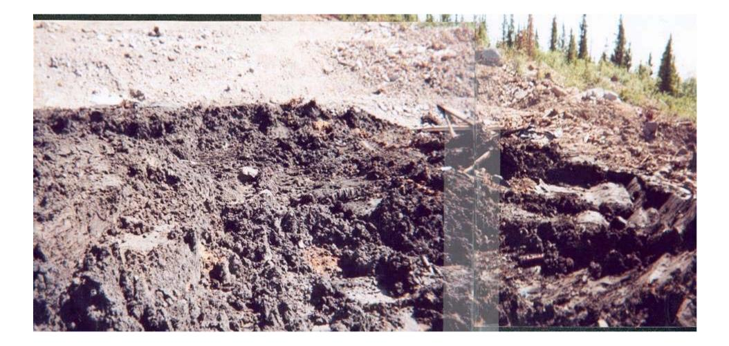
A decision was made to attempt to pit mix the remaining material rather than try to sort out the debris The QA/QC was handled by determining the remaining quantity and applying the stabilizer to the pit en masse.
