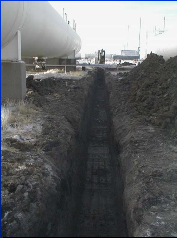
Excavation of Collection Trench
